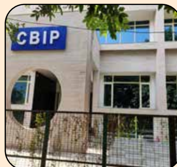
CBIP Centre of Excellence at Gurgaon (2020 onwards) Sector 32, Plot No. 09
