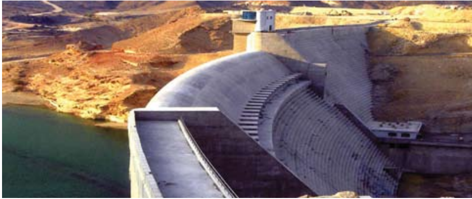
Figure 5 : View of Dayqah Dam from the left abutment (taken from RMD, 2014).
