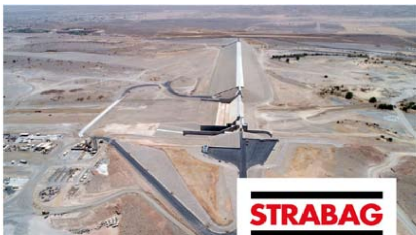
Figure 7 : Aerial view of Fulajj Dam (taken from STRABAG, 2017).
