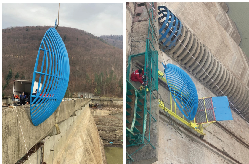
Figure. 7 : The new trash rack
