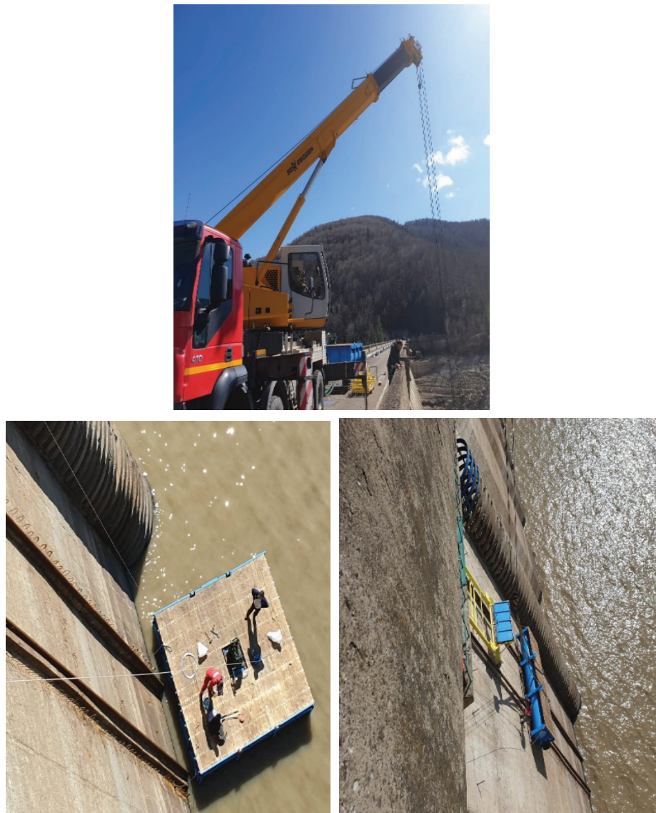
Figure 3 : Placing of the working pontoon on the water
