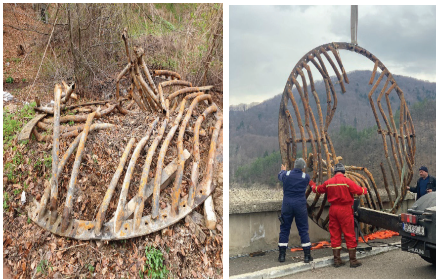
Figure 6 : Remains of the old trash rack
