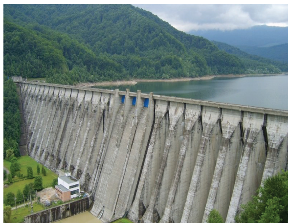
Fig. 1 : View of Poiana Uzului Dam from the downstream left abutment
