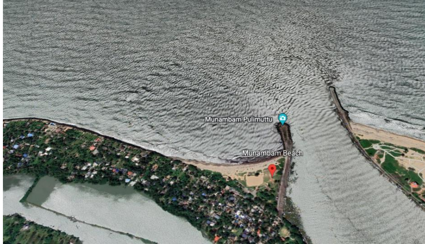
EyeROV Inspection Services
