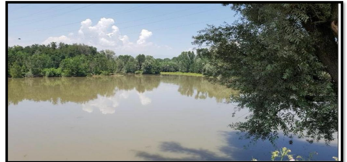
Jhelum Out Fall Channel Silted up due to Pohru Nallah.
