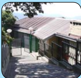
CBIP Office at Shimla (1927-1952)
