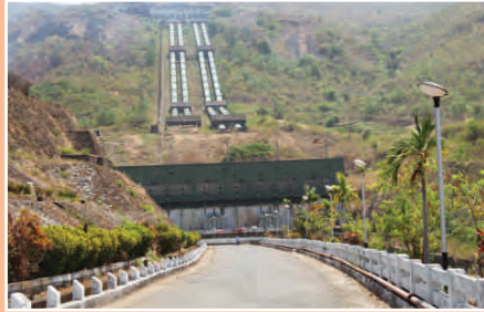
Upper Kolab Hydro Electric Project, Bariniput, Odisha
