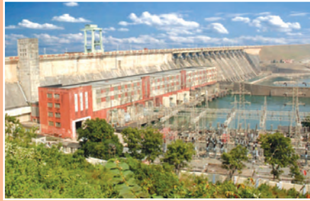
Hirakud Hydro Electric Project, Burla, Odisha
