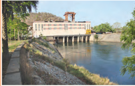
Chiplima Hydro Electric Project, Chiplima, Odisha
