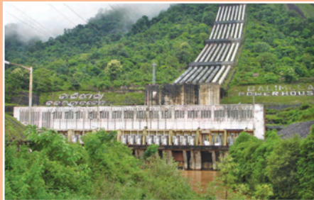
Balimela Hydro Electric Project, Balimela, Odisha
