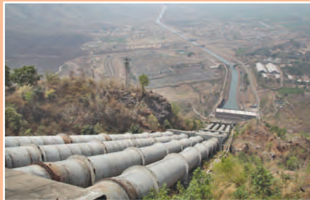
Upper Indravati Hydro Electric Project, Mukhiguda, Odisha
